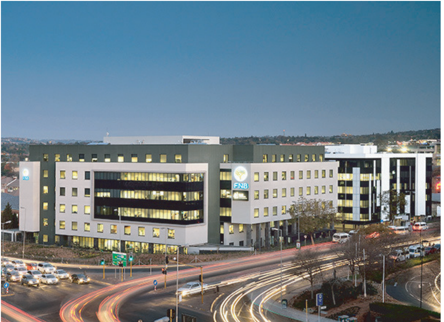
FNB Menlyn Corner – Supplied grilles, weather louvres and fans
